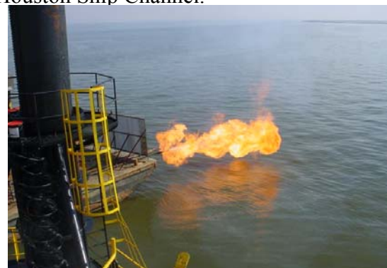
Photograph 2 (View of flare/vent line from the well)
