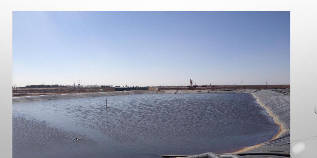
And finally the water is pulled out of the storage pit and pumped to the well site to be used in the fracturing process.
