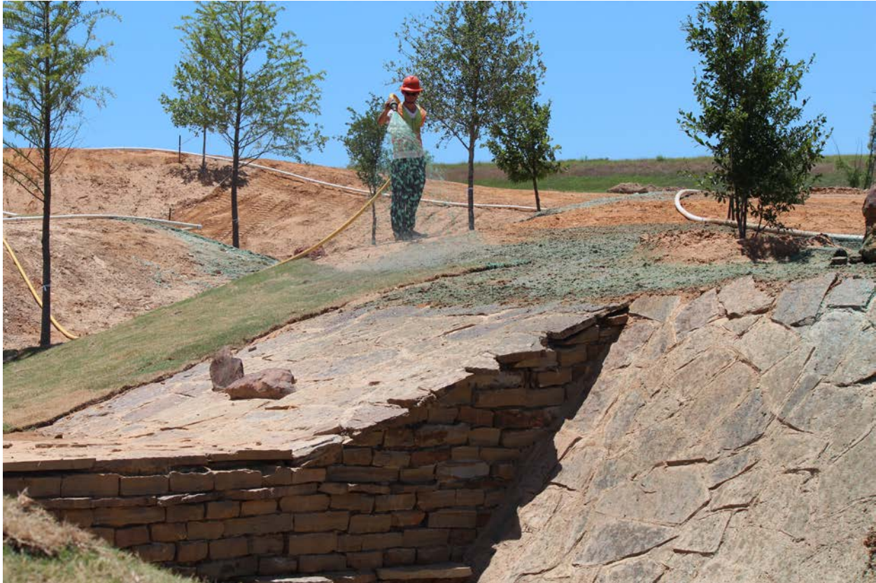
Figure No. 2 – Applying hydro mulch near the middle vertical drop structure.
