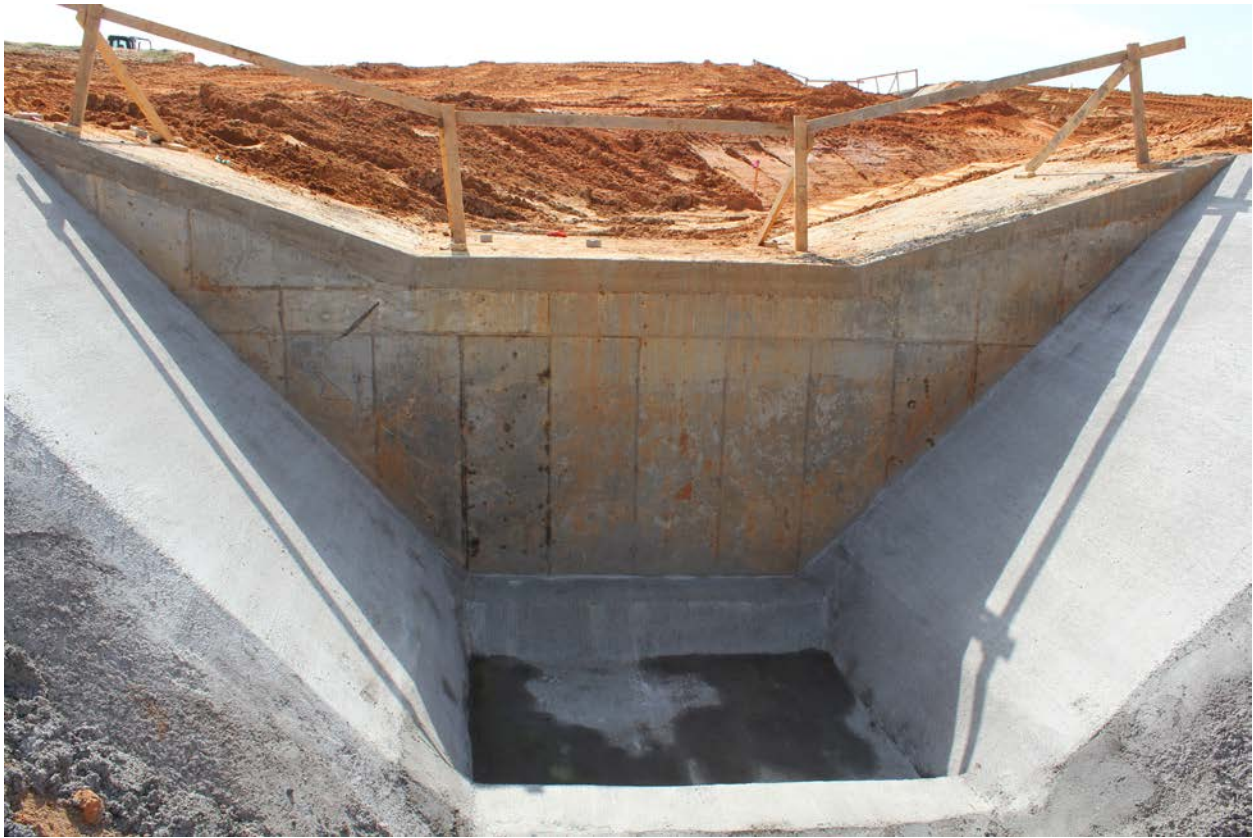
Figure No. 1 – Final concrete construction of the middle vertical drop structure.
