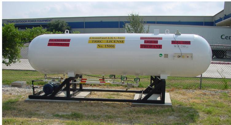
Figure 11. Supply Container, Pump and Bypass
