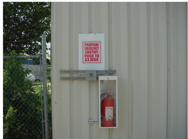
Figure 13. Emergency Shutdown Station and Fire Extinguisher
