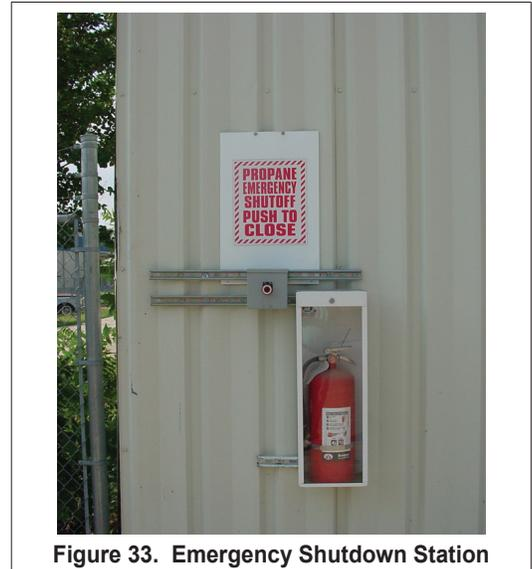
Figure 33. Emergency Shutdown Station
