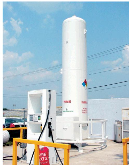
Figure 18. Vertical Tank, Single-Vehicle Dispenser and Meter/Control Unit
