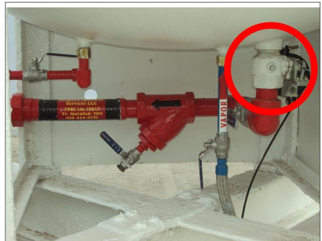
Figure 25. Internal Valve With Automatic Shutoff
