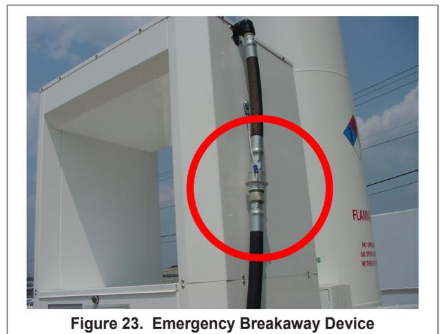
Figure 23. Emergency Breakaway Device
