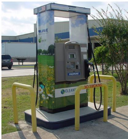
Figure 12. Dispenser Meter and Control Unit
